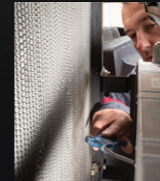
Plenty of room to access radiators for cleaning.
